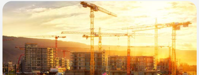
CONSTRUCTION, REMEDIATION, DEMOLITION
